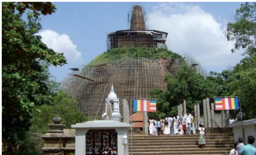
The Abhayagiri undergoing restoration works
